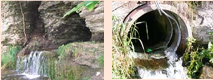
Figure 2. Subsurface hydrologic features in Sny Magill and South Fork watersheds. In the Sny Magill watershed (left photo), springs and caves discharge natural drainage from unknown areas of karst terrain. In the South Fork watershed, once-prevalent wetlands were converted to cropland with tile drainage. This 36-inch clay pipe (right photo) has discharged drainage collected from about 4,500 acres of cropland for nearly 100 years (note monitoring lines).
